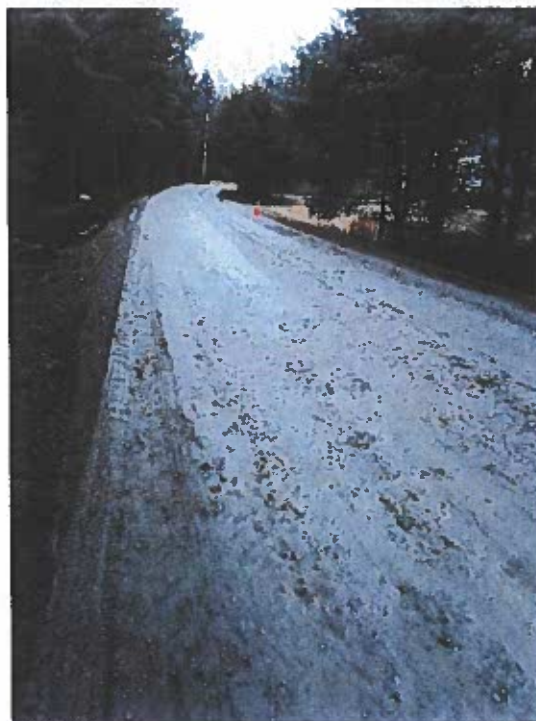
Picture 23 – Insufficient roadway surface
