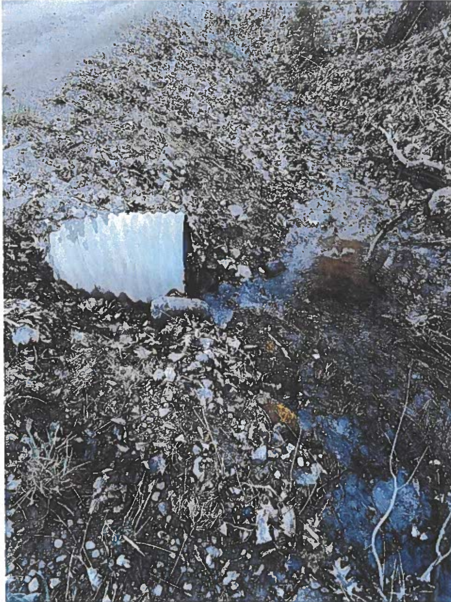
Picture 12 – 24" HDP Culvert
