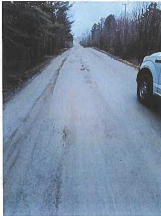
Picture 4 – Insufficient roadway surface and/or poor roadway aggregate
