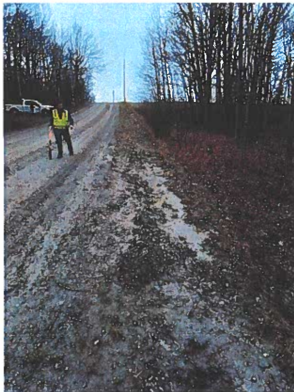
Picture 1 – False Ditch on southern side of roadway
