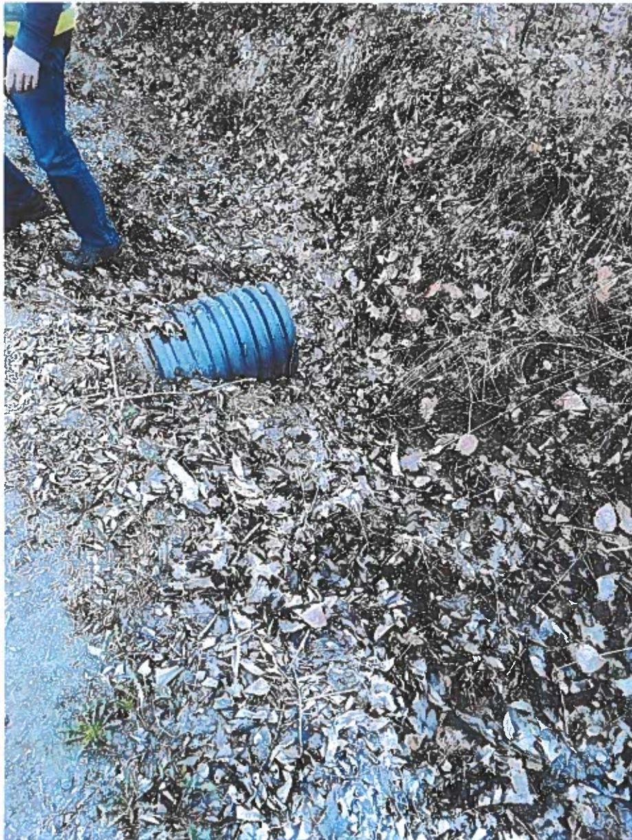
Picture 13 – 24" HDP Culvert
