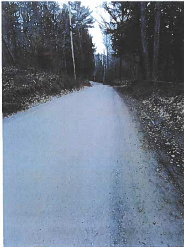
Picture 19 – Ditching Required
